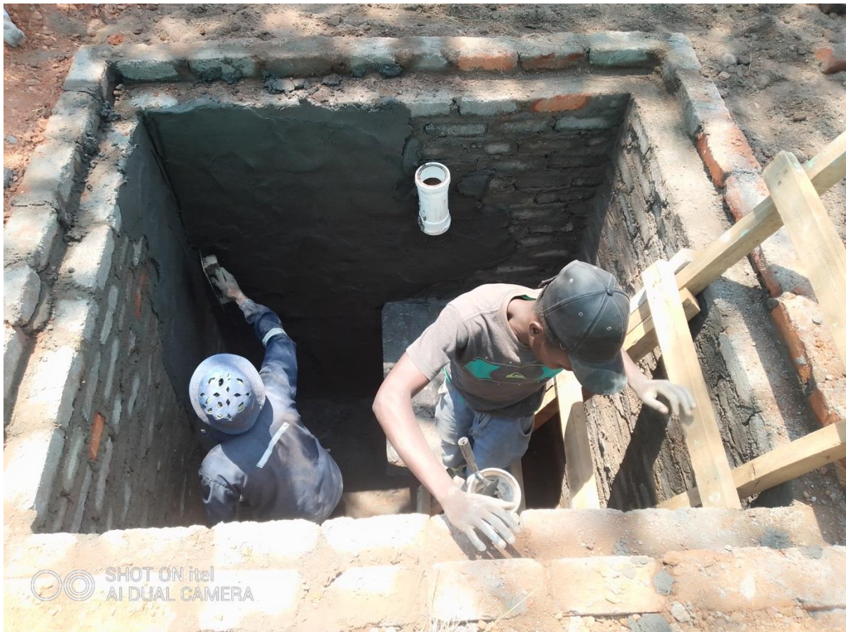
The septic tank under construction
